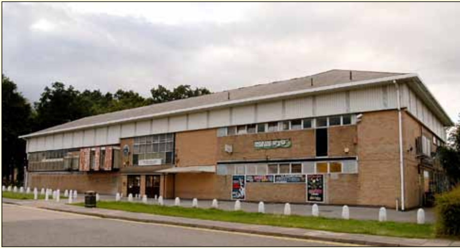
The New Parks Club is one of the biggest in the Midlands and one of the most prominent buildings on the New Parks estate.
